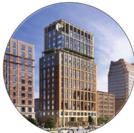
The Apsley Status: Completed City: New York, NY 142 units
